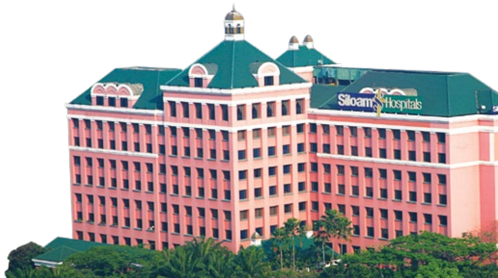
Siloam Hospitals Lippo Village, Indonesia
