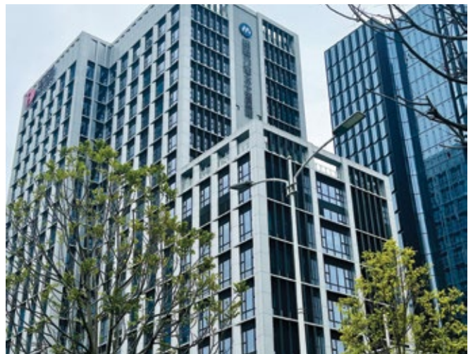
Exterior facade of Prince Bay Hospital in Shenzhen, China
